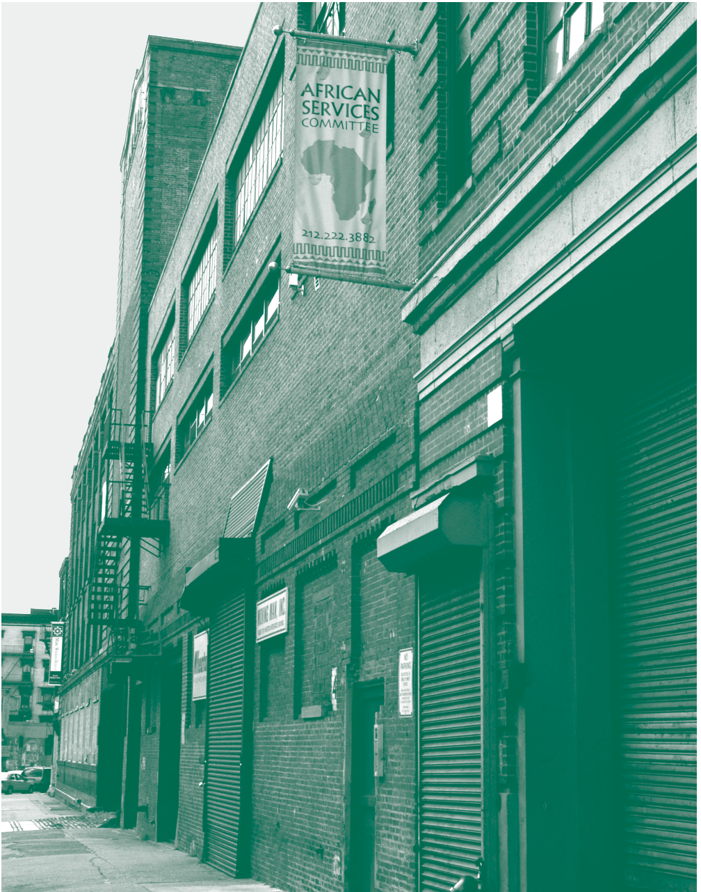
Establishing a strong foundation in Harlem with the expansion of our office space at 429 West 127th Street in New York City. Photo by Jake Price.
